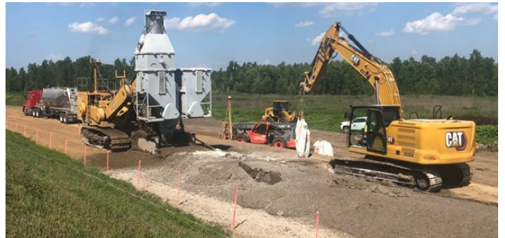
Figure 10: Waconda Lake Dike and Levee emergency design repairs
